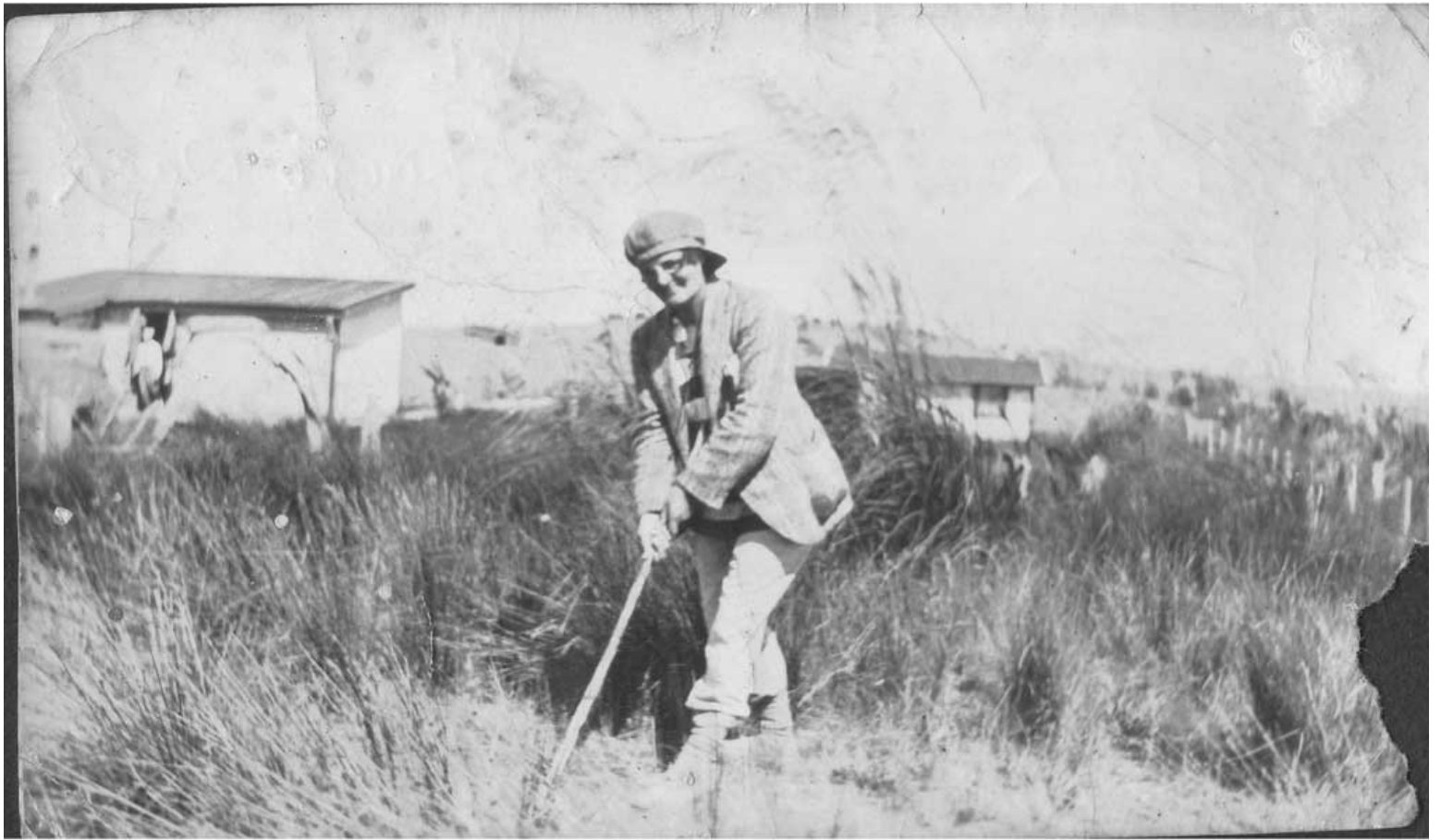
Above: 1920's: Looking towards the sea from the Omanu street area, the bach on left is at 25 and on right at 27 Rapaki street.
