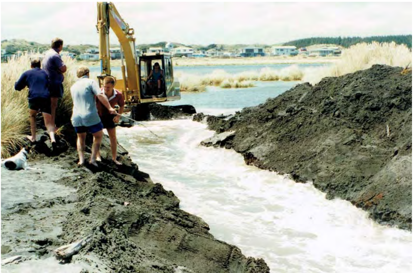
1997: Second attempt to drain the water.
