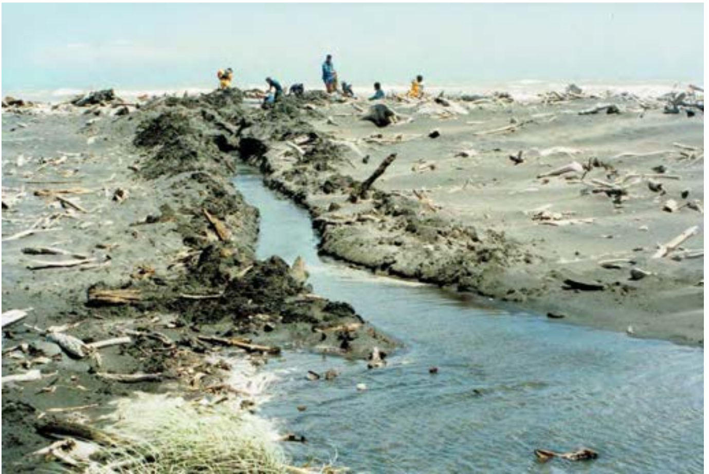
1997: First attempt to drain the water.
