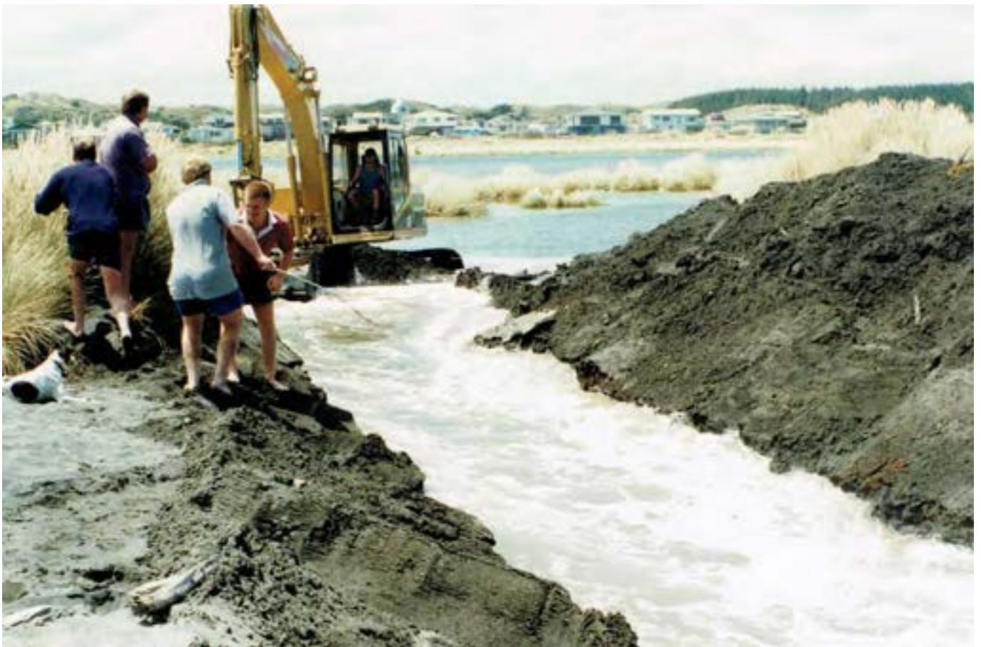
1997: Second attempt to drain the water.
